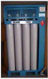
Aluminum cylinders are lightweight but are temperature sensitive, In a fire they can rupture due to heat embrittlement
