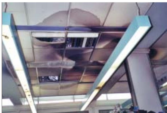
Flood-damaged ceiling.
