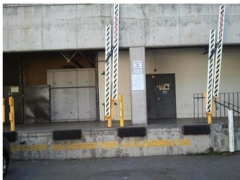
Safety warning rails should be in the up or open position only during loading operations.
