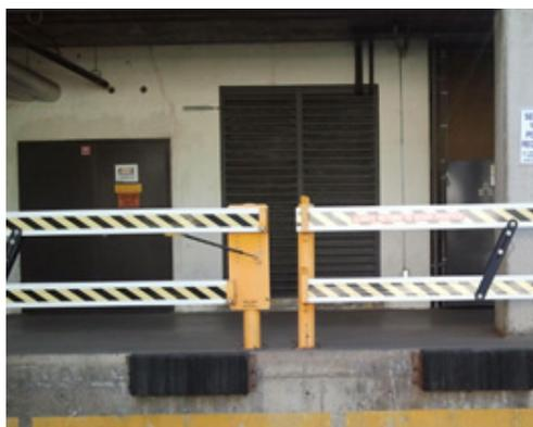
Keep rails down when loading is not in progress.
