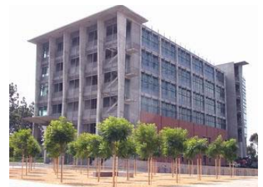
Buildings with outdoor stairs are great for fresh air exercise and taking in the view.
